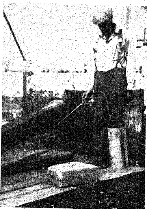
Figure 76. Oiling a poorly constructed cesspool that breeds mosquitoes
